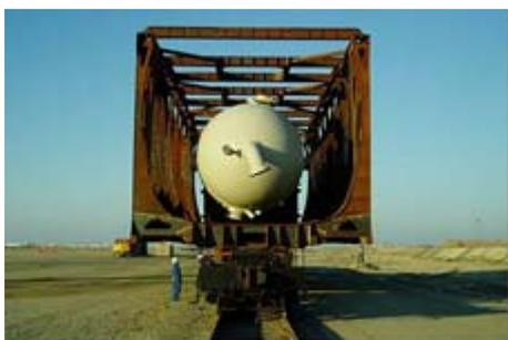
At every step of the journey, the scale of the effort matched the size of the equipment. At Aktau's port, for instance, it took 1,200-ton cranes to safely hoist the cargo off the barges and onto multiwheeled, multi-axle carriers.
