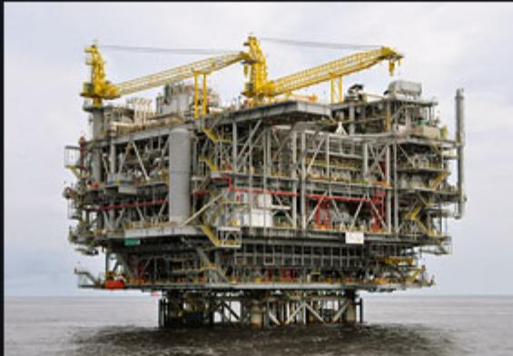
In 2009, we announced first oil from compliant tower development Tombua Landana, situated offshore Angola in about 1,200 feet (366 m) of water and standing at about 1,554 feet (474 m) – one of the world's tallest man-made structures.
