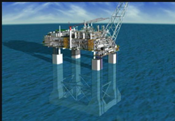
In their search for stronger fixed structures, facilities engineers also are taking a fresh look at gravity-based structures. Typically made with concrete (example: Hibernia, designed to withstand icebergs), Chevron plans to develop one made of steel, as shown here, for our Wheatstone platform offshore Western Australia. Steel was chosen to handle the region's unique, loose "calcarenite" soil.
