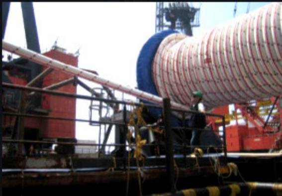
Traditional mooring lines that tether a structure to the sea floor are chain or steel-wire rope, fine for shallower water. But as you go deeper, those metal moorings become heavy, impinging on the buoyancy of the platform above and offsetting the floater - which is why we turned to polyester. Chevron is an industry leader for the number of polyester lines in deployment.
