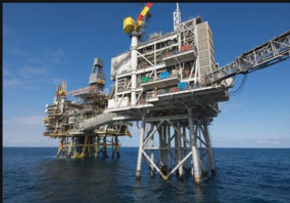
The Britannia Platform, jointly operated with ConocoPhillips, is located 130 miles (209 km) northeast of Aberdeen in the U.K. sector of the North Sea. It's a fixed drilling and production platform that sits in about 492 feet (150 m) of water.
