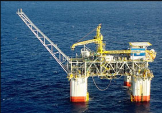
Blind Faith in the deepwater U.S. Gulf of Mexico is one of the industry's deepest semis, hitting the seabed nearly 6,500 feet (1,981 m) below the surface.
