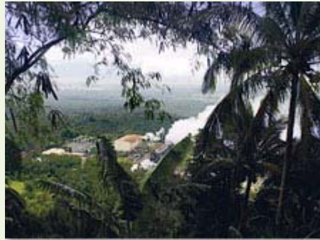
In the Philippines, the Mak-Ban (seen here) and Tiwi plants produce geothermal energy to supply 7 percent of the electricity required by Luzon island’s 43 million people.
