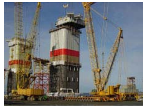
Blind Faith hull construction at Aker Kaverner fabrication yard in Norway.
